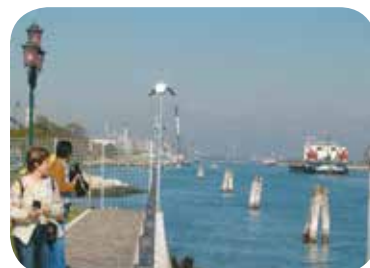
SL-125-C lanterns installed at marina, Venice, Italy
